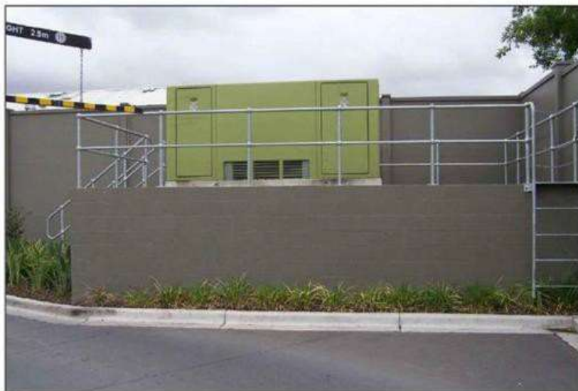
Figure 51 - Example substation raised above 1:100 flood level
